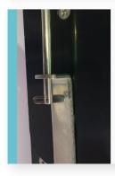
Ensure the drop nose end is correctly orientated to stop the pin working out.
